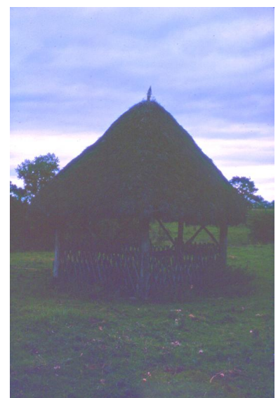
A general view of the well, taken by Eric Dunstall in late summer 1966
