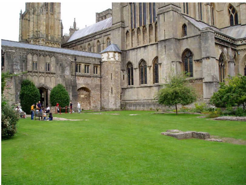
Left: A view from the south across, and approximately at right angles to the place where the English foundations lie.
